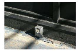
4.15 - SAFETY: We strongly recommend that the receptacle in any bathroom, exterior, or wet location be protected with ground fault circuit interrupters.
