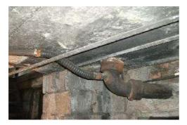
5.7 - DEFICIENT: The fixture drain on the basement sink was not properly installed and vented. Please contact a licensed plumber to repair in accordance with local code requirements or to move the sink to another location. The current sink is draining on to the floor surface drain.
