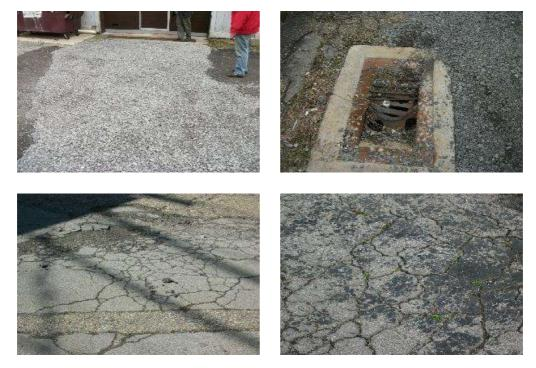
1.7 - DEFICIENT: The asphalt driveway is functional but has some cracks and areas needing repairs.
