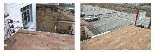
4.3 - SAFETY: The overhead conductor lines to the garage are too low and need to be raised by the utility company.
